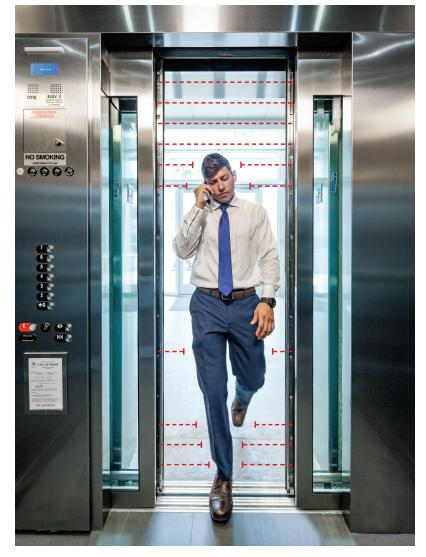
The Optiguard door protection system utilizes 154 infrared beams to continuously scan for interruptions. If any beam is interrupted, the Optiguard system will instantly reopen the elevator door.
